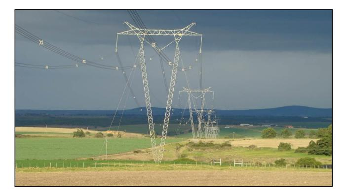
**Plate 6**: View along Alternative 2 indicating the impacts of the existing 400Kv 520 Guyed Vee towers and line on the undulating countryside.
